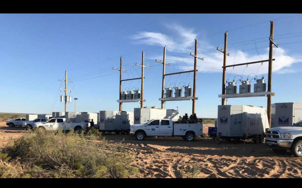
For five years, Mesa Natural Gas Solutions has been manufacturing generators that can run on the natural gas associated with oil production. Half the company's business is in the Permian Basin.
